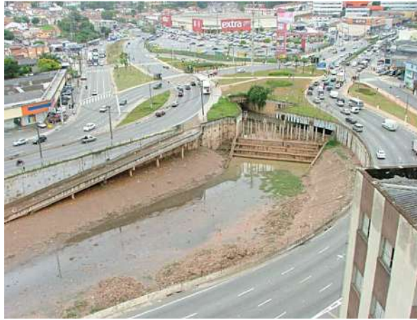
Figure 8 A detention reservoir in Sao Paulo that is used for flood control (Moura et al., 2015, p. 247)
